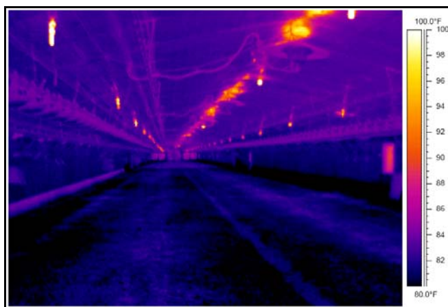
Figure 4. Thermal image of house using side wall inlets between flocks (summertime).
